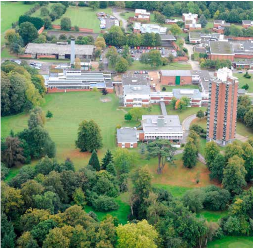
Aerial View of Wilton Park former Defence School of Languages, from the North
