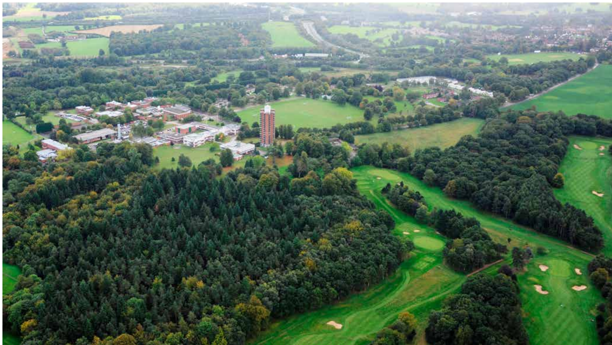
Aerial view of Wilton Park Opportunity Site
